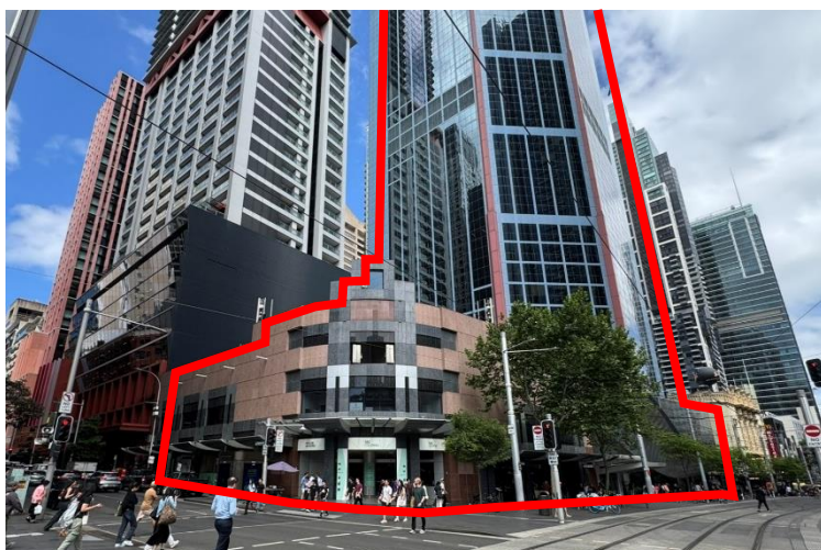
Figure 2: Looking south-east toward the subject site (in red)
